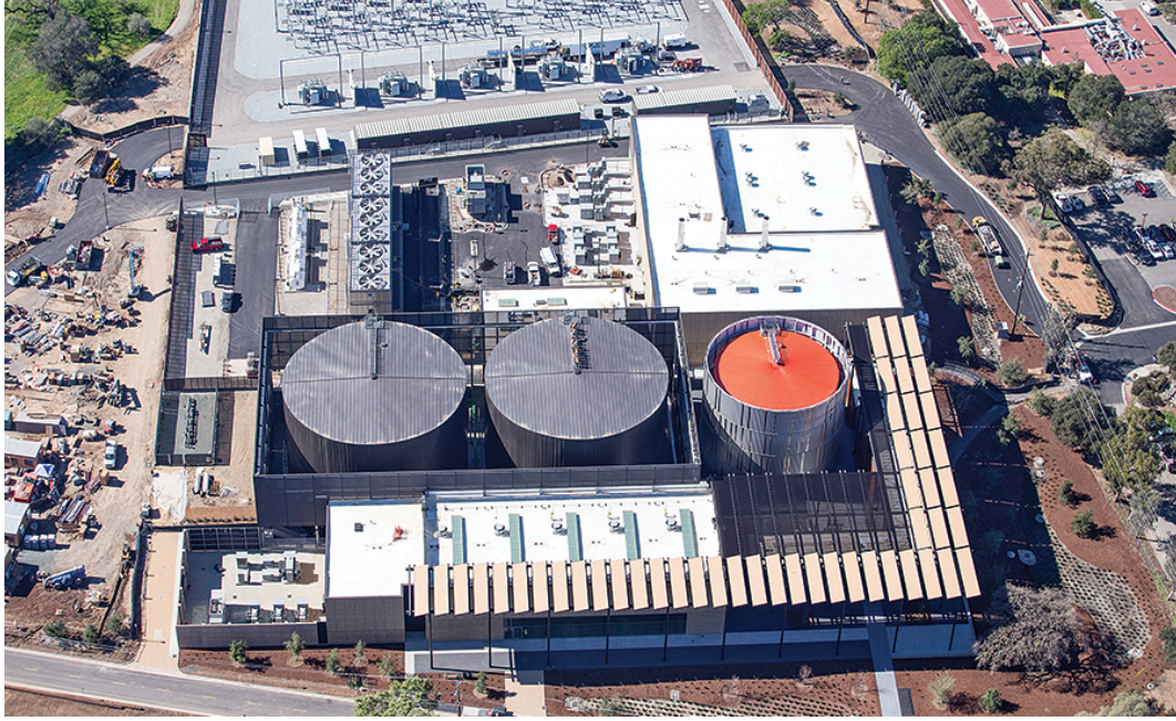
Figure 1: The new heat-recovery system to provide heating and cooling to the campus constructed as part of the $485-million Stanford Energy System Innovations (SESI) project Blair (2016).
